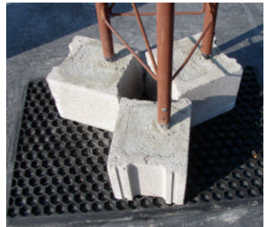
10' tower, guyed, socket: 3 cement blocks on a rubber mat
