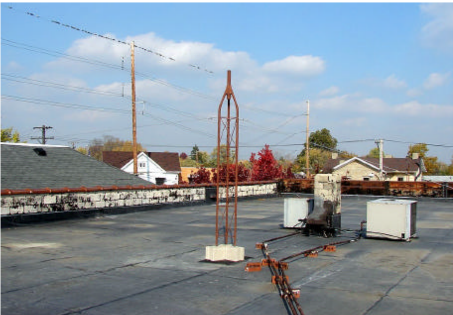
10' tower, guyed, socket: 3 cement blocks on a rubber mat
