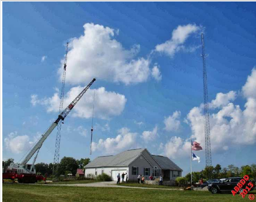
Matt's, K7ND, new towers, self supporting, one 100', the other 140'
