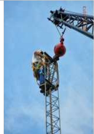
^^^Climbing up to disconnect the crane.^^^
